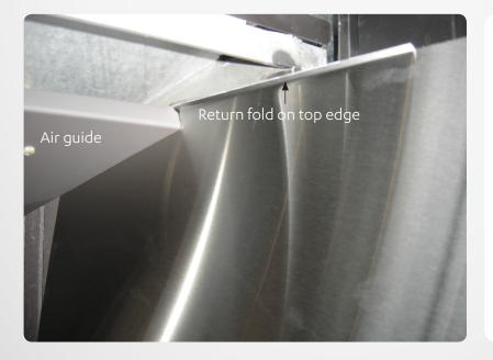
Slide the panel into place by positioning the return fold on the top edge of the panel on top of the air guide, it will drop down slightly (approx. 12 mm). This will keep the panel suspended in place.
