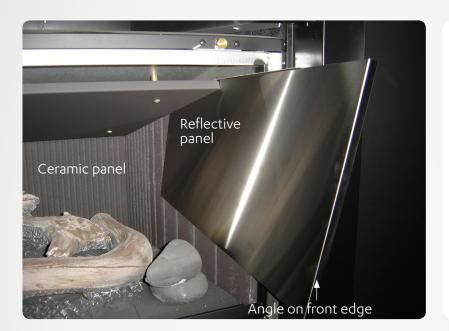
The reflective panels are designed to slide in and cover the existing ceramic panels. The ceramic panels remain in place inside the unit.
