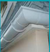
Fit Downpipe brackets at 2 metre spacings for vertical pipes and 1.2 metres for graded pipes.
